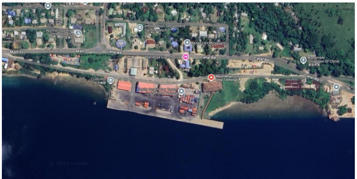
Figure 2: Luganville Wharf is large enough for powerful warships to dock Source: Created by the Author using Google Earth
